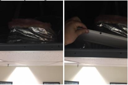
• There is no air flow off VAV-41 and 42A. This is due to a possible bad VAV controller.
