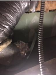
• Drop number two off VAV-53 had no air flow. This is due to the ceiling diffuser being placed on top of ceiling tile.
