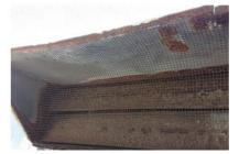
The overall condition of the fan is poor. There are holes from corrosion throughout the unit. The dampers for the economizer and outside air are corroded. The insulation from inside the fan compartment is coming off the unit walls and the fan itself is dirty and needs to be cleaned.
