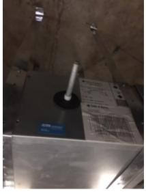
• Air Distribution 9, 10, 12 and 13 have an actual CFM of 0. On 9,10 and 12 that is due to the ductwork not being installed properly on the ceiling diffuser and possibly blowing above the ceiling. Drop 13 has no air flow due to the duct work not being connected.
