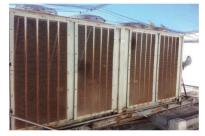
Due to deterioration and rusted shut dampers and shafts, the air distribution system does not provide the code necessary ventilation air required for space comfort.
