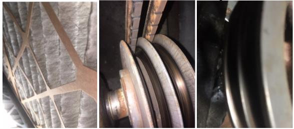
• The coils on the unit have minor corrosion on them along with damaged fins. Cleaning these coils and repairing the fins will increase performance and air quality.
