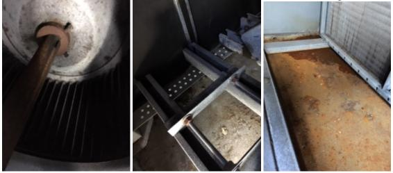
• The supply duct work has damage to it which is leaking air. Sealing this duct work will insure that it will reach the conditioned space.
