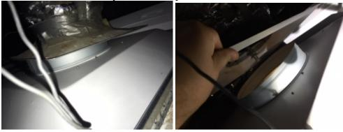
• Air Distribution 7,9 and 10 associated with VAV-30 have an actual CFM of 0. This is due to the diffuser being capped.
