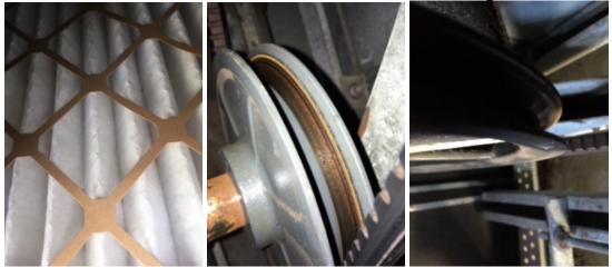
The coils on the unit have minor corrosion on them along with damaged fins. Cleaning • these coils and repairing the fins will increase performance and air quality.
