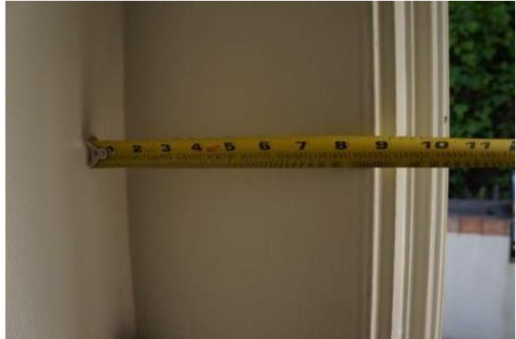
Photo 13. Example of a door that does not comply with the California Building Code.
