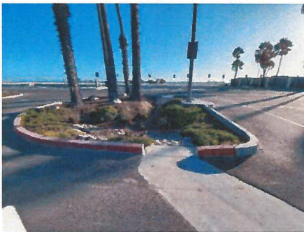
Figure 8: Bioretention/infiltration facilities.
