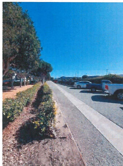
Figure 4: Concrete swale within public parking lot.
