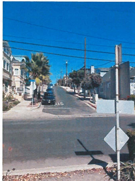
Figure 3: Typical City cross gutter.
