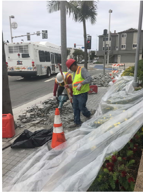
Preparation Work— Removal of gray tiles
