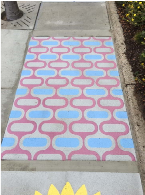
Geometric Thermoplastic over smooth concrete
