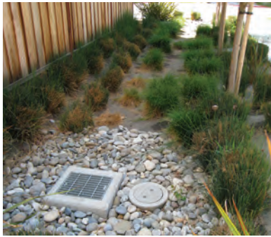
Figure 25 Vegetated bioswale filters stormwater
