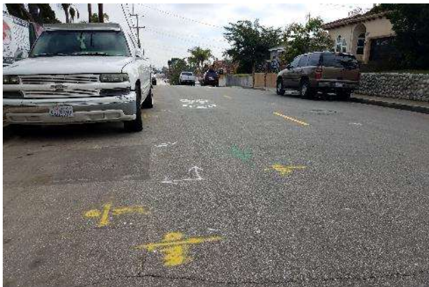
PHOTO 1: USA MARKINGS SHOWING LOCATION OF EXISTING UNDERGROUND UTILITIES ON 2 ND ST (LOCATION S-G7)
