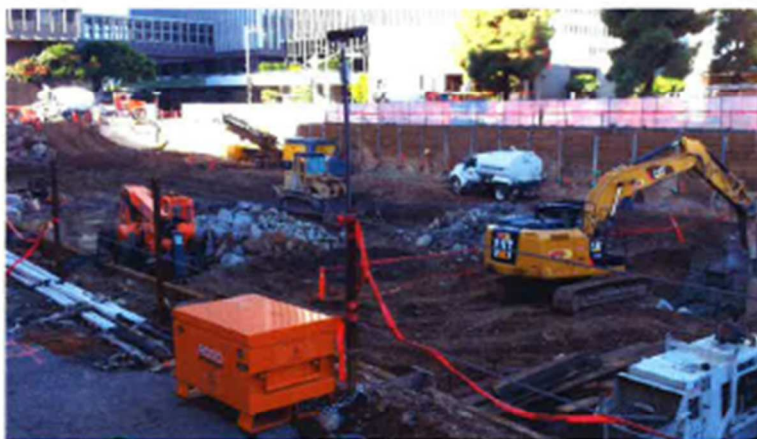
Figure 1: GEOVision vibration monitoring system at a DTLA site. Includes cellular remote email alarm and warning strobe.
