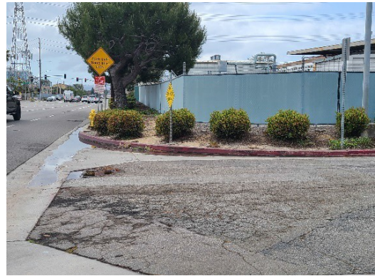
Distressed asphalt pavement to be replaced with wide PCC cross-gutter
