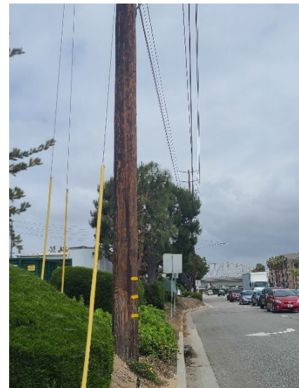
SCE power poles and guy wire obstruction through proposed sidewalk alignment
