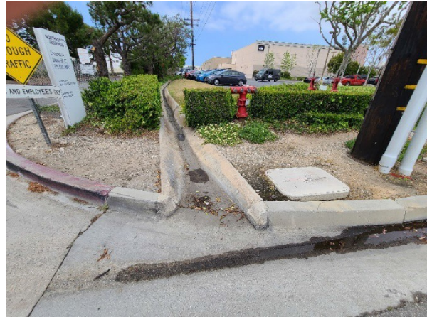
Flow from storm water culverts to be diverted through sidewalk outlet structures
