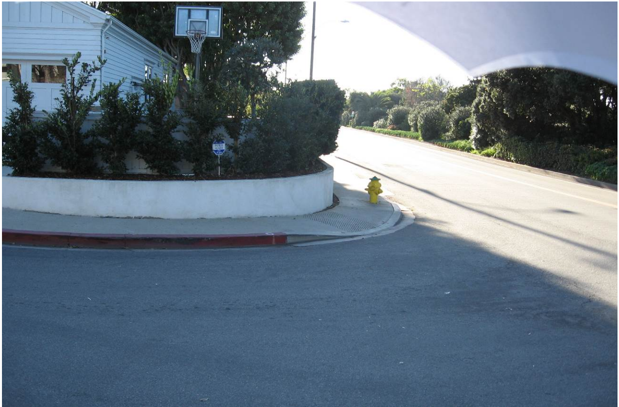
Southwest Corner of Ardmore Avenue at Flournoy Road (Bushes Overhanging Sidewalk)
