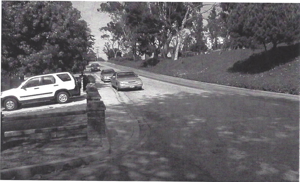
Valley Drive at Flournoy Avenue Looking East
