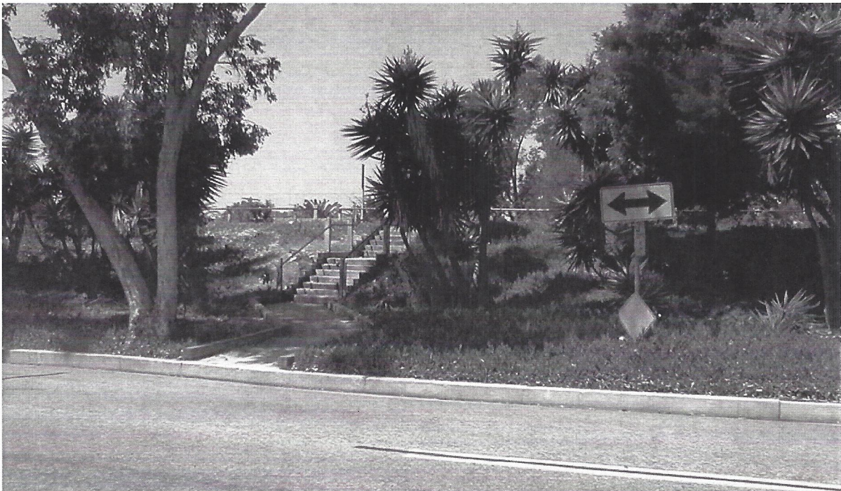
Access Path to Veterans Parkway at Ardmore Avenue/Flournoy Road
