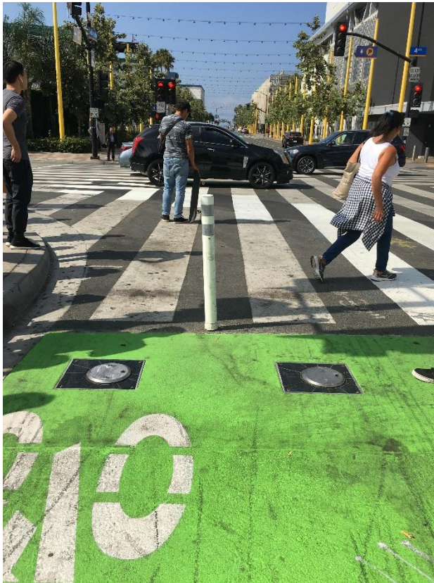
8-inch assistant retractable bollards, crash rated
