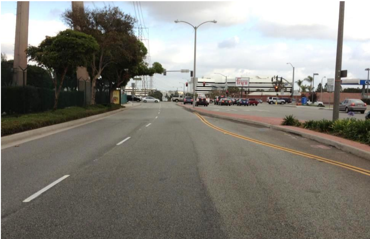
Westbound Rosecrans Avenue at Elm Avenue Looking East
