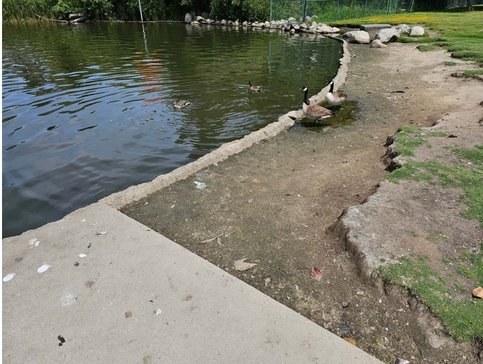
Photo 1. The southern end of the pond is ringed with bare soil outside of the concrete rim for a segment of 60 feet. This muddy area can develop puddles used by geese and other wildlife.
