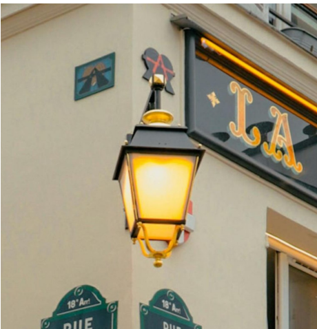
Code compliant light fixtures are allowed with appropriate permits
