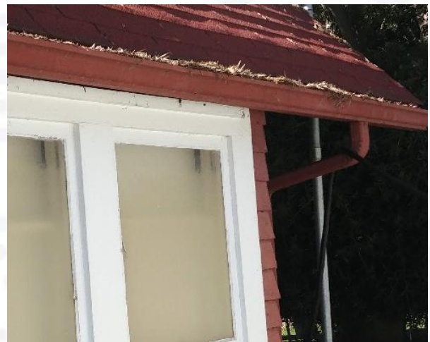
Figure 22: Run gutters of the beach cottage overflowing with dead leaves
