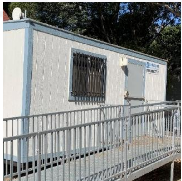
Figure 28: Trailer's security features bars on the window and a lock-bar
