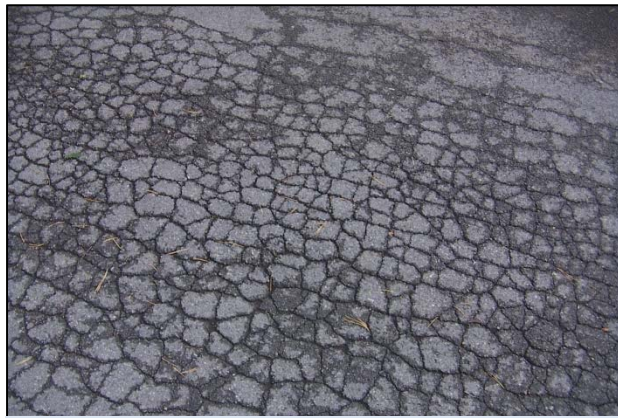
Alligator Cracking
