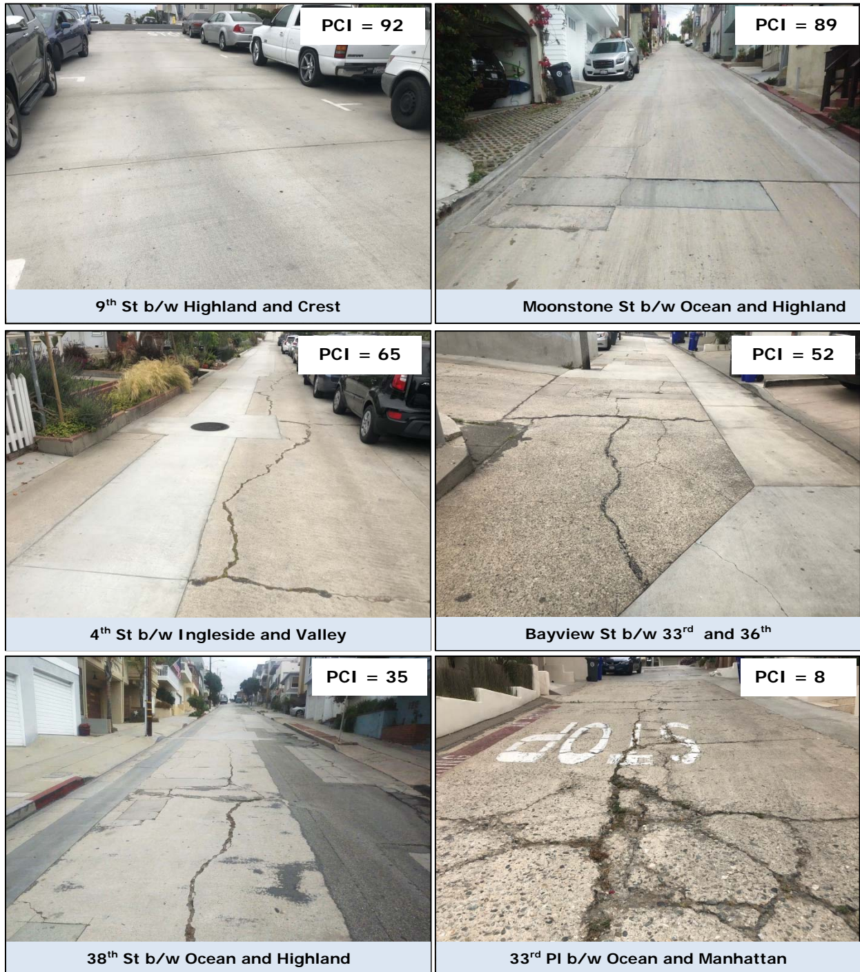
Figure 5: Examples of PCC Streets with Different PCIs
