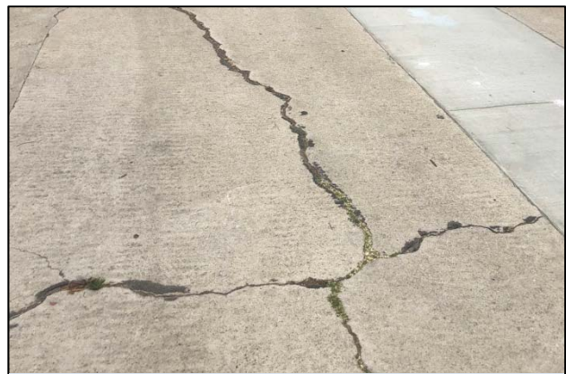
Linear Cracking
