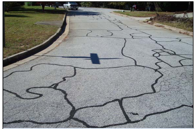
Block Cracking
