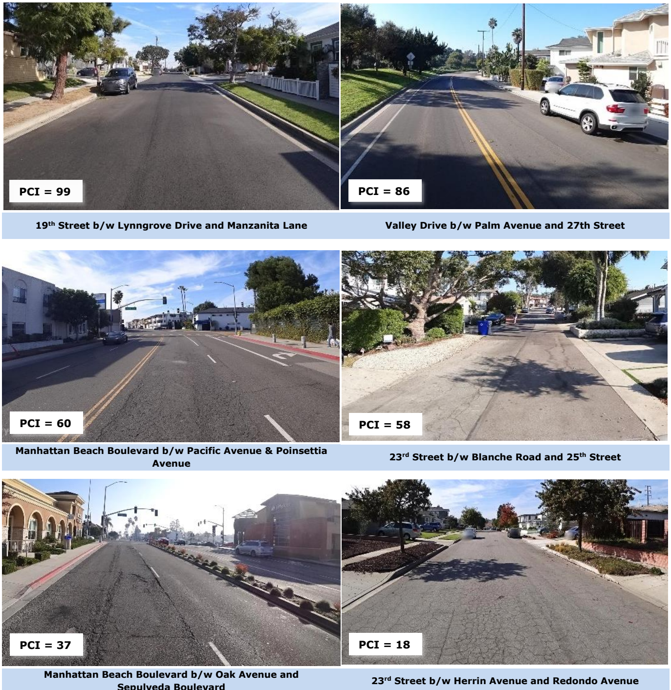
Figure 4: Examples of AC Streets with Different PCIs
