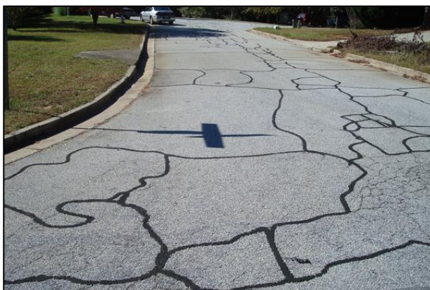
Block Cracking
