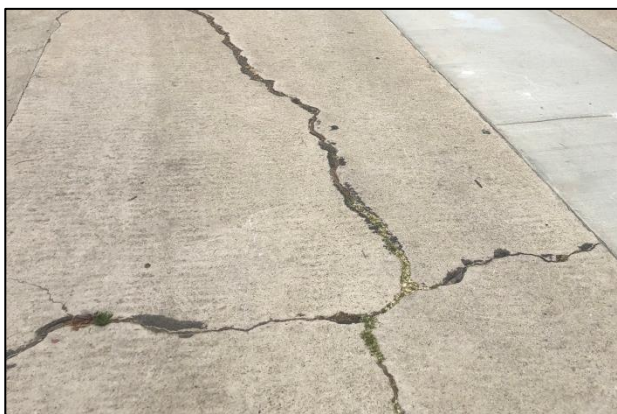
Linear Cracking
