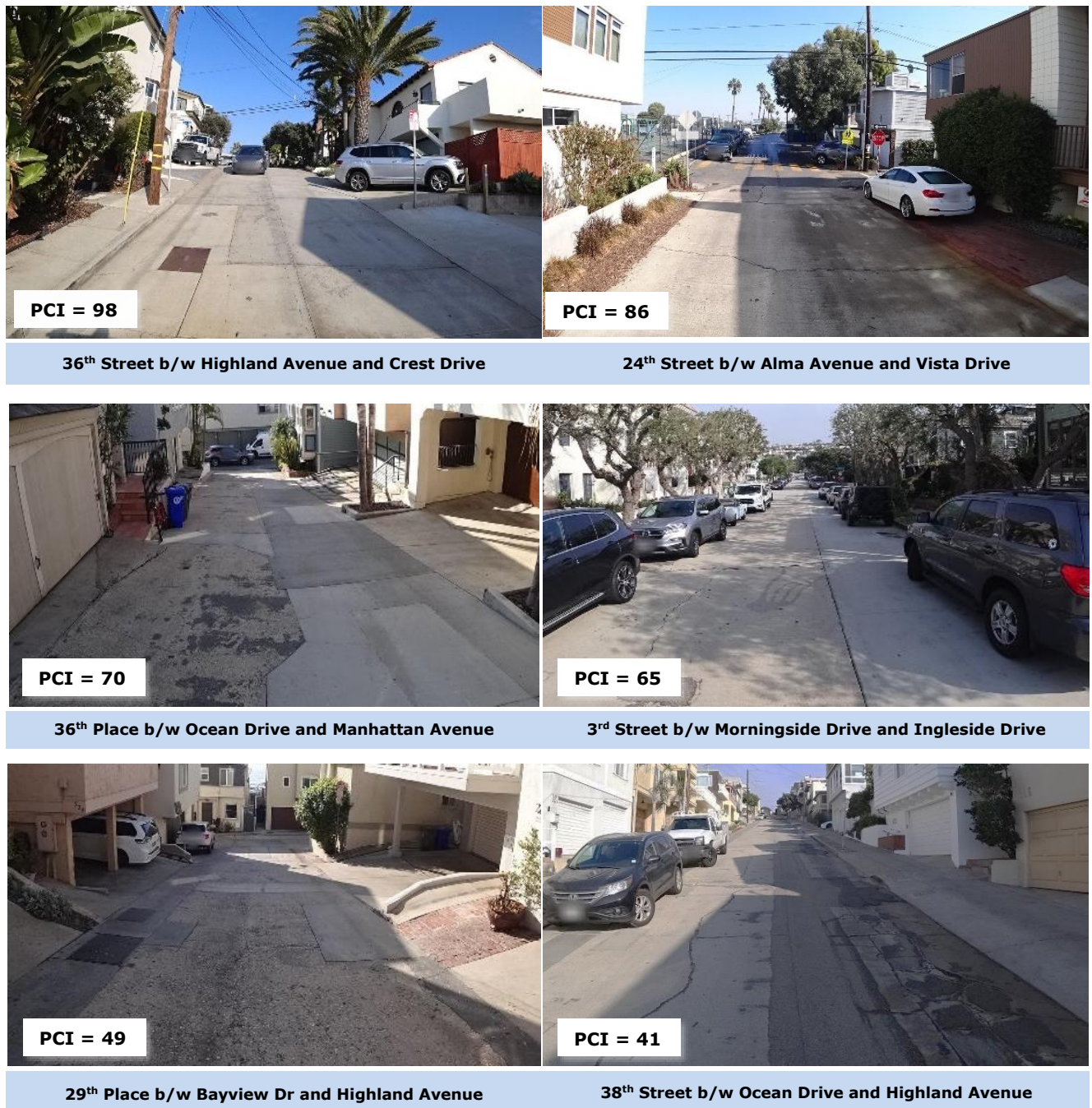
Figure 5: Examples of PCC Streets with Different PCIs
