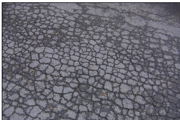
Alligator Cracking
