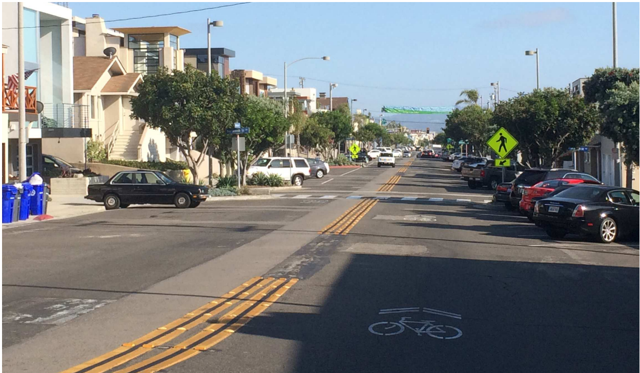
Manhattan Avenue at 15 th Street Looking South After
