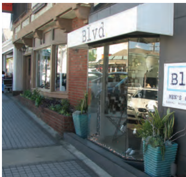
Figure 9 Transparent windows along ground-floor retail
