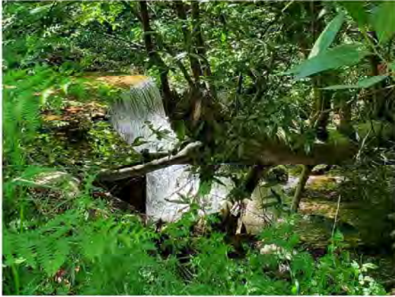
Figure 4-1. Concrete Box Structure
