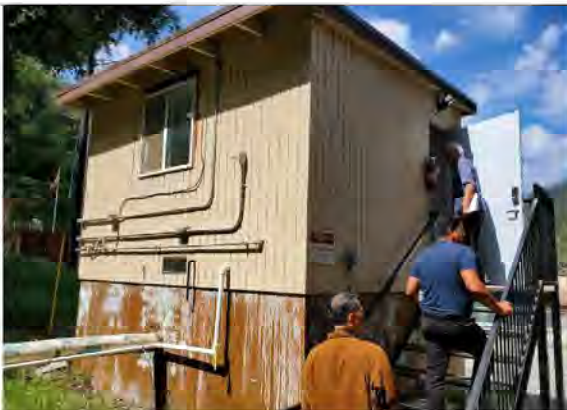
Figure 4-2. Clearwell / Pump House
