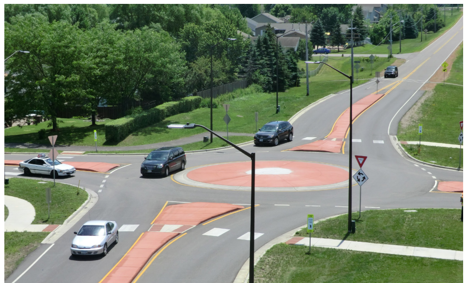
Example of a single-lane roundabout. Source: FHWA
