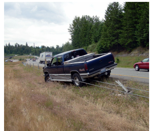
Median cable barrier prevents a potential head-on crash. Source: Washington State DOT
