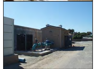
Equipping of Well No. 31
