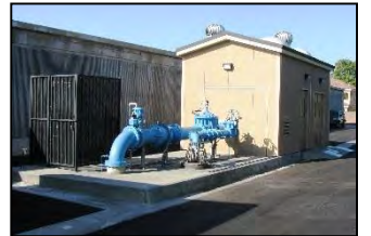
Equipping of Well 31 and Lampson Reservoir Booster Pump Station Upgrades
