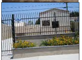
Myra Avenue In-Line Detention Basin and Stormwater Pump Station No. 2
