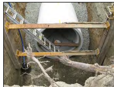
Electric Avenue Storm Drain
