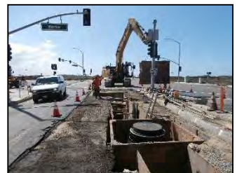
Warner Avenue Gravity Sewer
