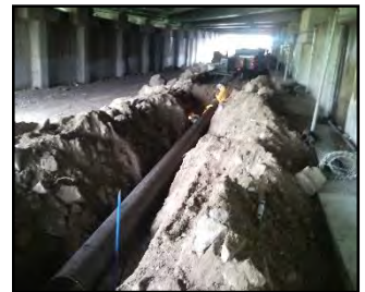
Pipeline Construction under I-5
