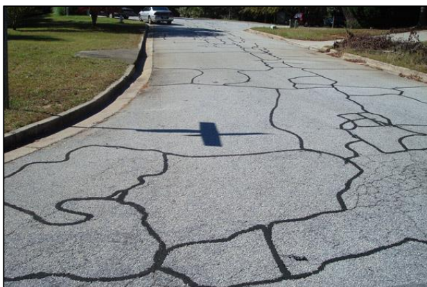
Block Cracking
