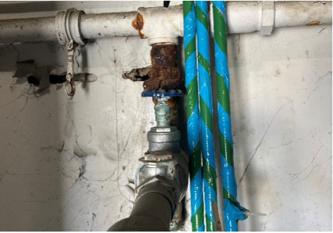
(FIGURE 4) EXAMPLE OF PIPE CORROSION
