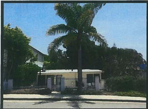
2. Front View (Ardmore Ave)
