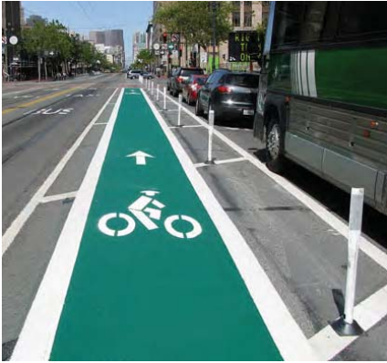
Green-colored bicycle lanes: San Francisco, CA (Credit: San Francisco Municipal Transportation Agency)
