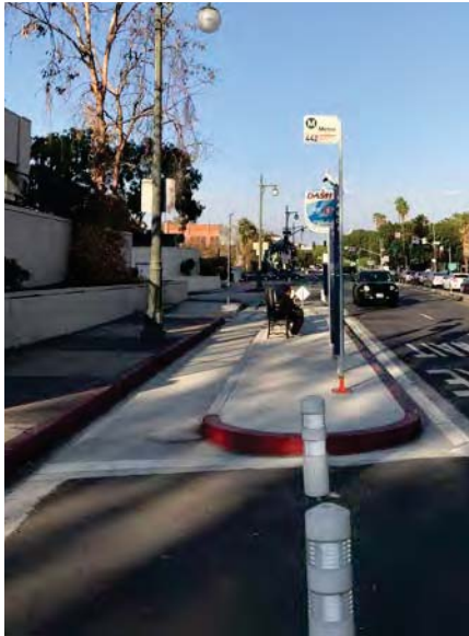
Bus stop islands should provide adequate space for bus stop amenities like seating and signage
