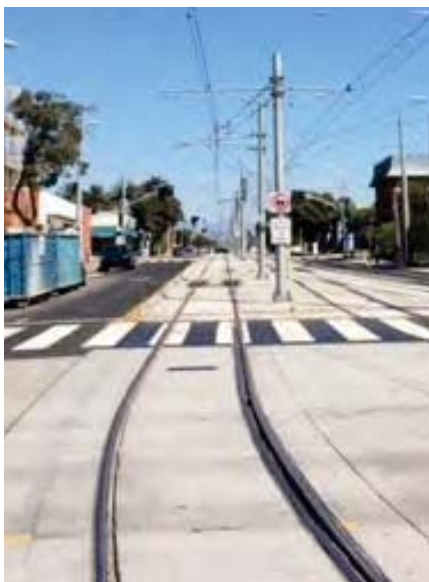
The gaps between rails and adjacent pavement at grade crossings, known as flangeways, can be hazardous to bicyclists and other users who rely on wheeled mobility devices
