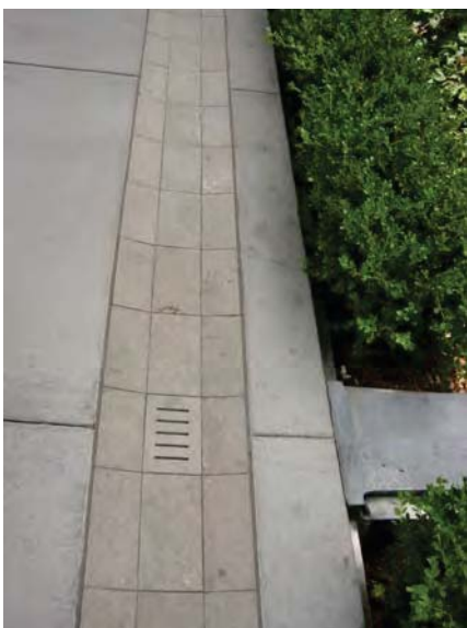
Constructed swale with drain (Credit: Stephanie Landregan)
