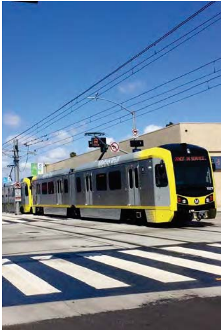
Light-rail in urban street: Santa Monica, CA
