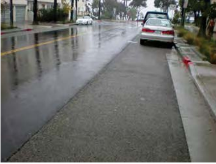
Permeable concrete after a rain event (Credit: Neil Shapiro)
