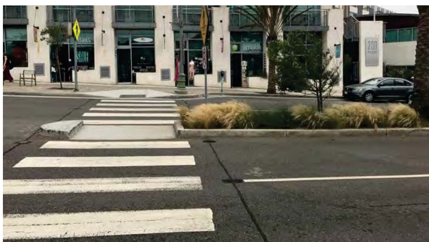
Curb extensions and a median make crossing four-lane streets safer and more manageable
