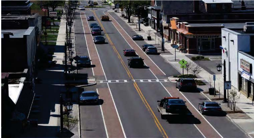
Parking assist lane (Credit: Michael Wallwork)
