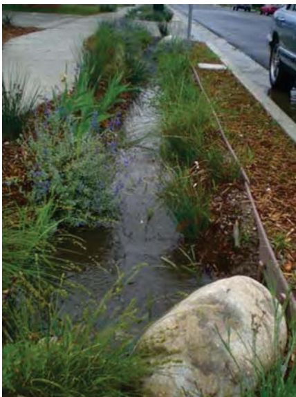
Sidewalk-adjacent swale during storm event (Credit: Edward Belden, Los Angeles and San Gabriel Rivers Watershed Council)
