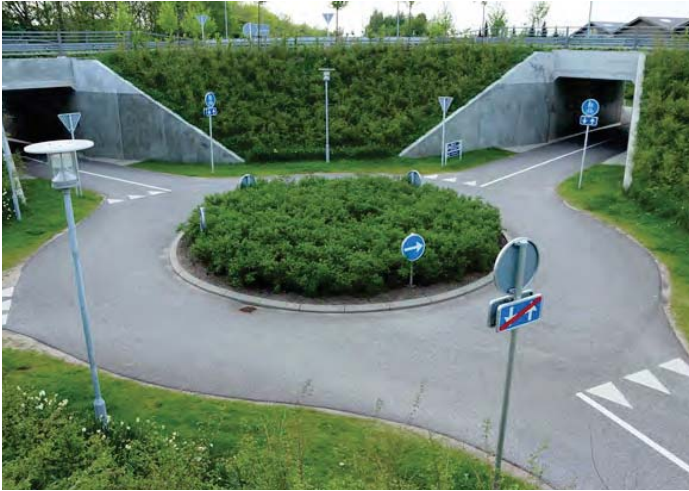
Left: Grade-separated intersection
