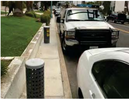
Narrow and obstructed sidewalk
