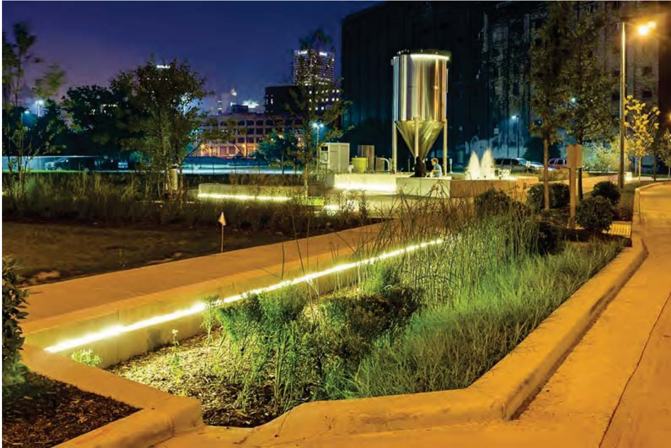
Mid-block curb extension with bioswale
