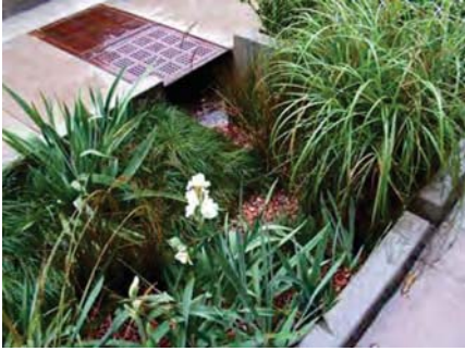
Swale with curb cut opening and decorative grate outlet (Credit: AHBE Landscape Architects)
