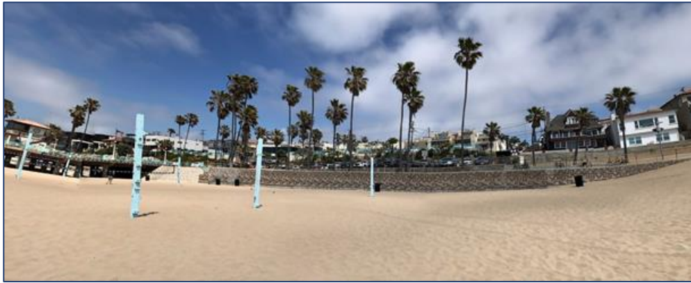
Existing Seawall MB Pier
