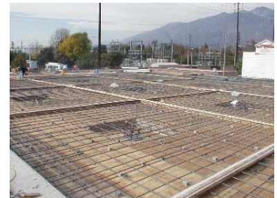
Typical Checkered Board Reservoir Roof Pattern
