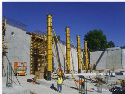
16.0 MG Evans Reservoir Construction
