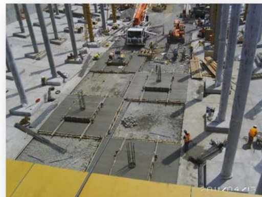
16.0 MG Evans Reservoir Construction
