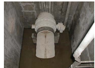
Reservoir Inlet Pipe Wall Penetration
