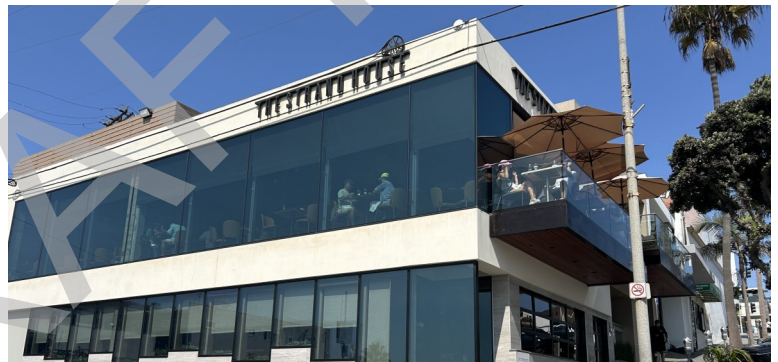
Existing balconies with outdoor dining cannot further expand into the right-of-way.
